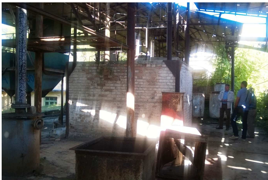
Photo 2. Refinery plant built before the Second World War, now is a museum object.
