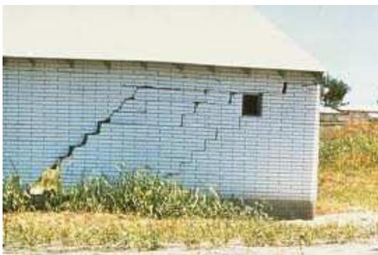
**Figure 1.** Damage of the school due to a sliding plane not evidenced before.
