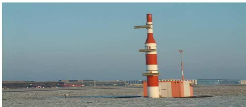
**Figure 4.** The UHF descent beacon draws a glide slope in the area
