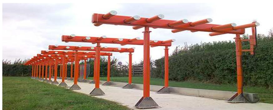
**Figure 2** Antennas of the localizer system
